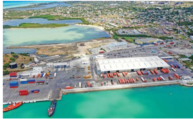
ABPA has invested in state-of-the-art cargo and logistics facilities
