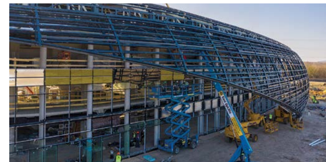
The construction of Tatabánya Multifunctional Sports Center
