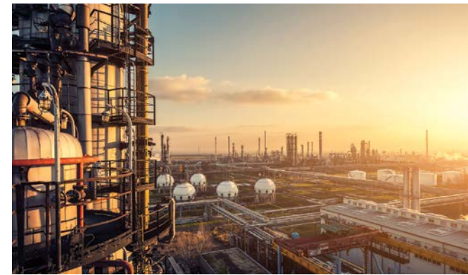
MOL's refineries are among the most efficient in Europe
