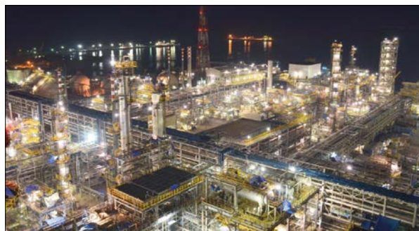
Petron Bataan Refinery.
