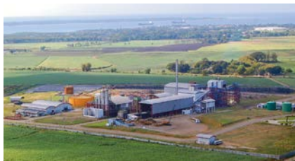
San Carlos BioEnergy Sugar, Ethanol and Power Plant
