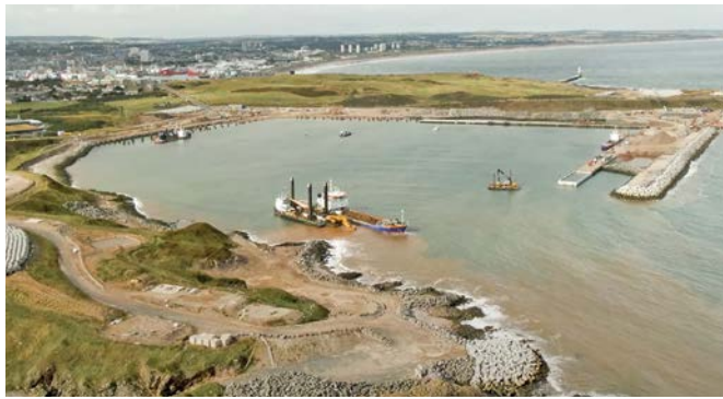
Aberdeen's new deep-water South Harbour
