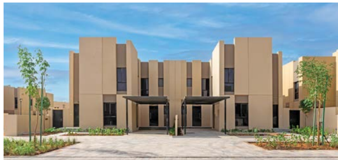
Saudi families have started moving into homes in SEDRA
