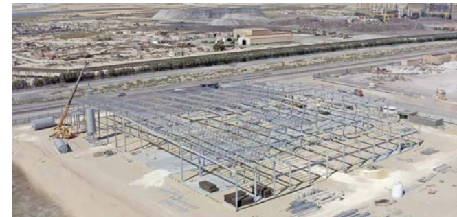
Gerflor Middle East's new 25,000m 2 rigid LVT plant
