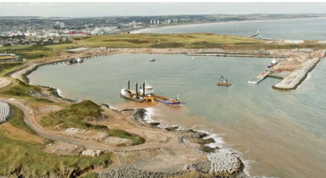
Aberdeen's new deep-water South Harbour
